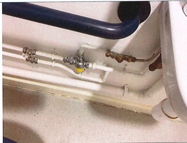
3. Example of in-line strainers
